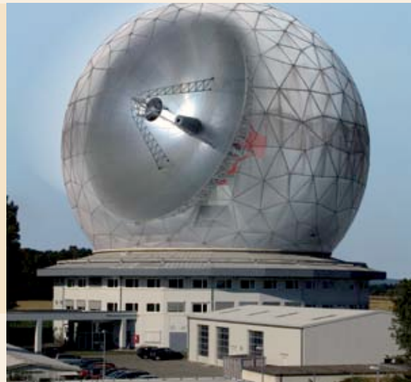
The Fraunhofer-Gesellschaft analyses space debris using the space observation radar system TIRA as well as other space objects, thereby contributing to safety in space.
